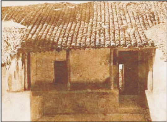
RAMANUJAN'S HOUSE IN KUMBakonam (~1900)
